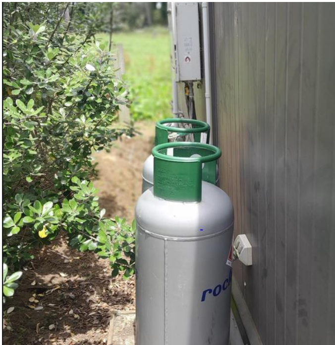
Figure 4– 90kg location not inspected by a certifier when certifying a >400 kg location at the same workplace
